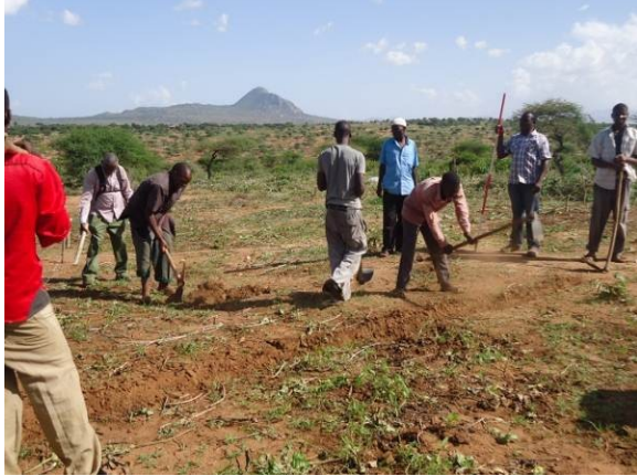
Pastoralists in Gairo district constructing the structures to conserve soil and water on their lands.
